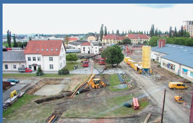
GRAZ - GBK BEFORE CONSTRUCTION WORKS
