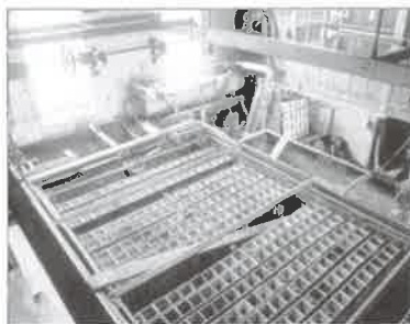
The room of the ponds, before demolition
