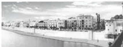
Right Bank: Patrocinio Bridge – Triana Bridge Section – Paseo de la O promenade
