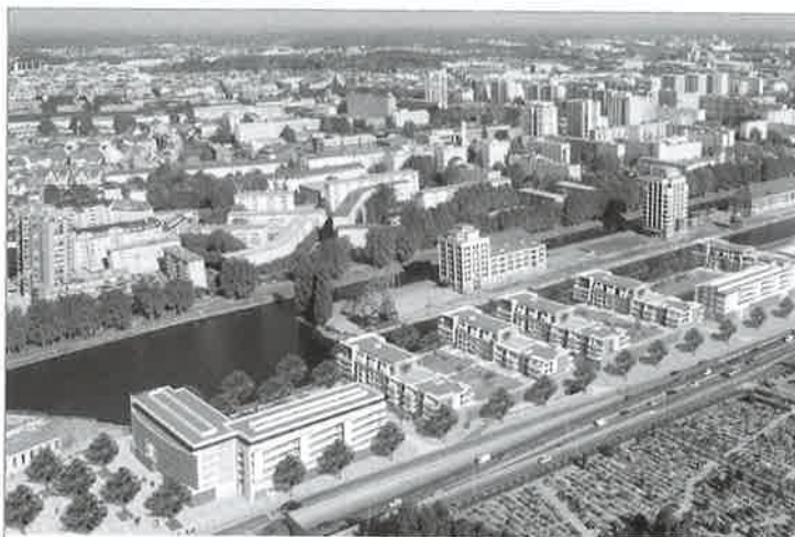
"Les passages de l'étoile" ["the passes of the Star"] (behind the former Austerlitz harbour), project management: SNC Passages de l'Etoile, SERS, Weller; architect: BIK,
